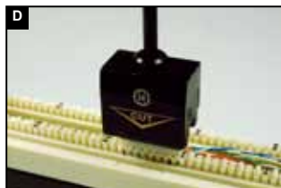
Install connecting block in the wiring block tightly.
