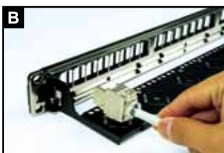
Position the shielded keystone jack for installation.
